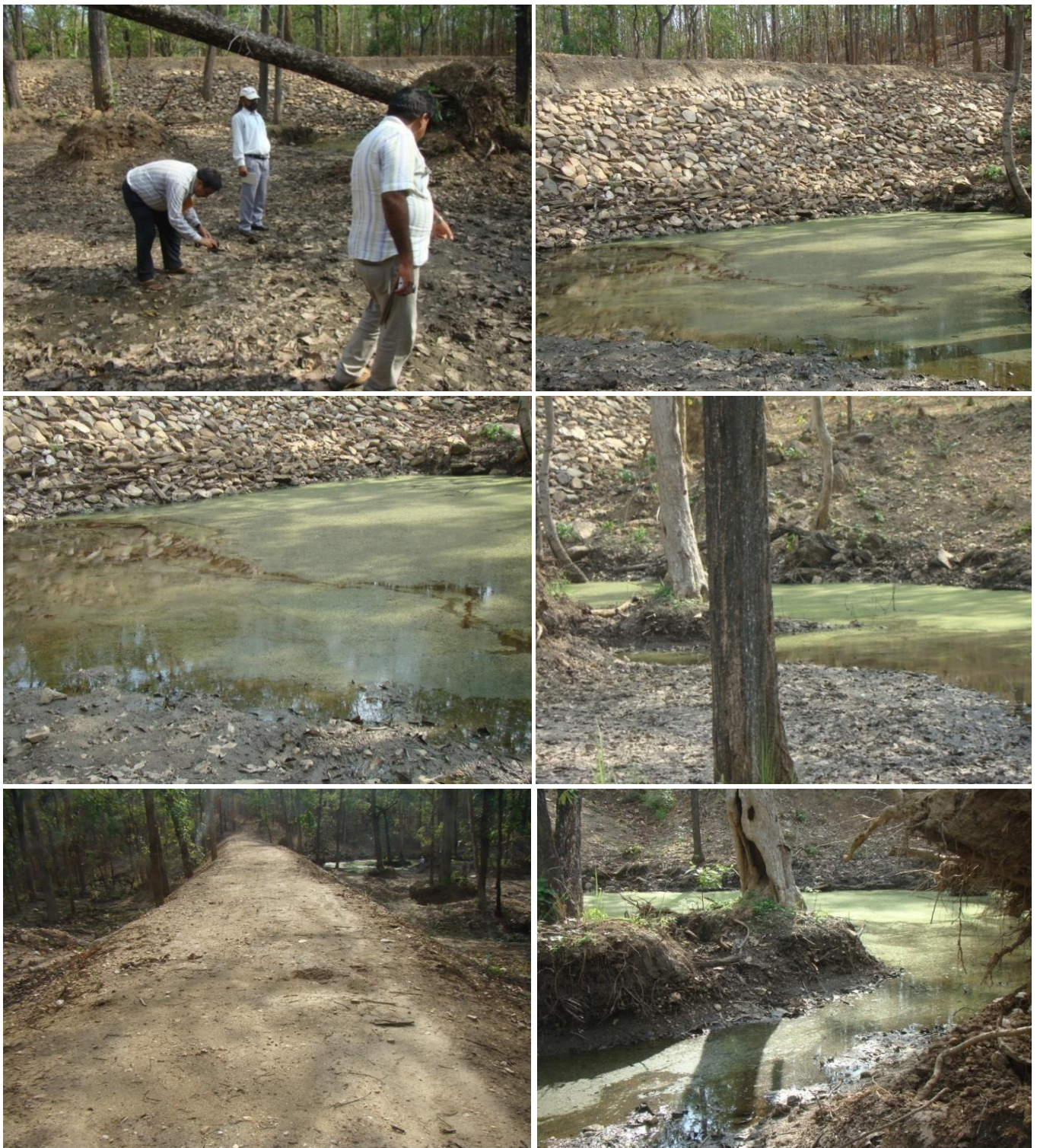
Fig. 3: Construction of check dam/pond - Site 2 (Photo dated 08.06.2016)
